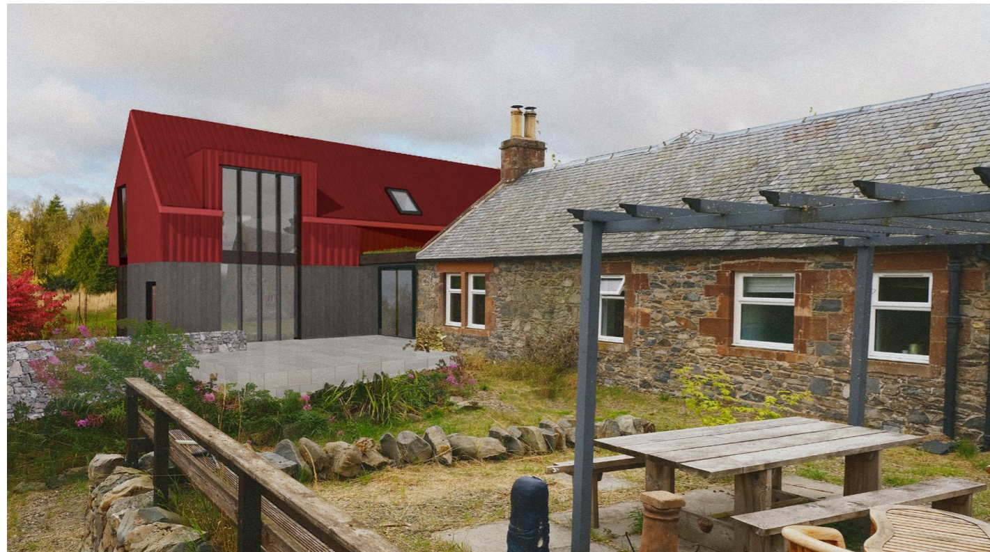
fig. 22 View of proposal from south east showing courtyard entrance to link building attached to west gable of the existing cottage.
